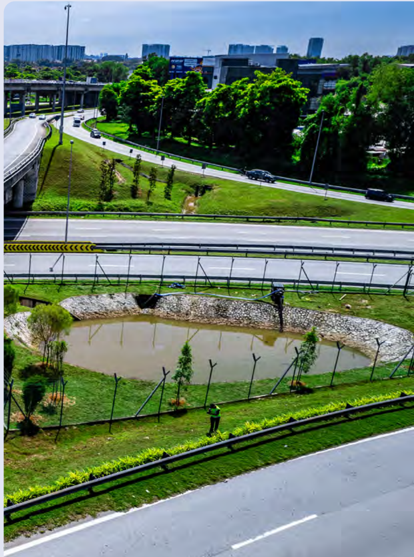
A retention pond along the GCE, supporting stormwater management, flood mitigation and a greener landscape.
